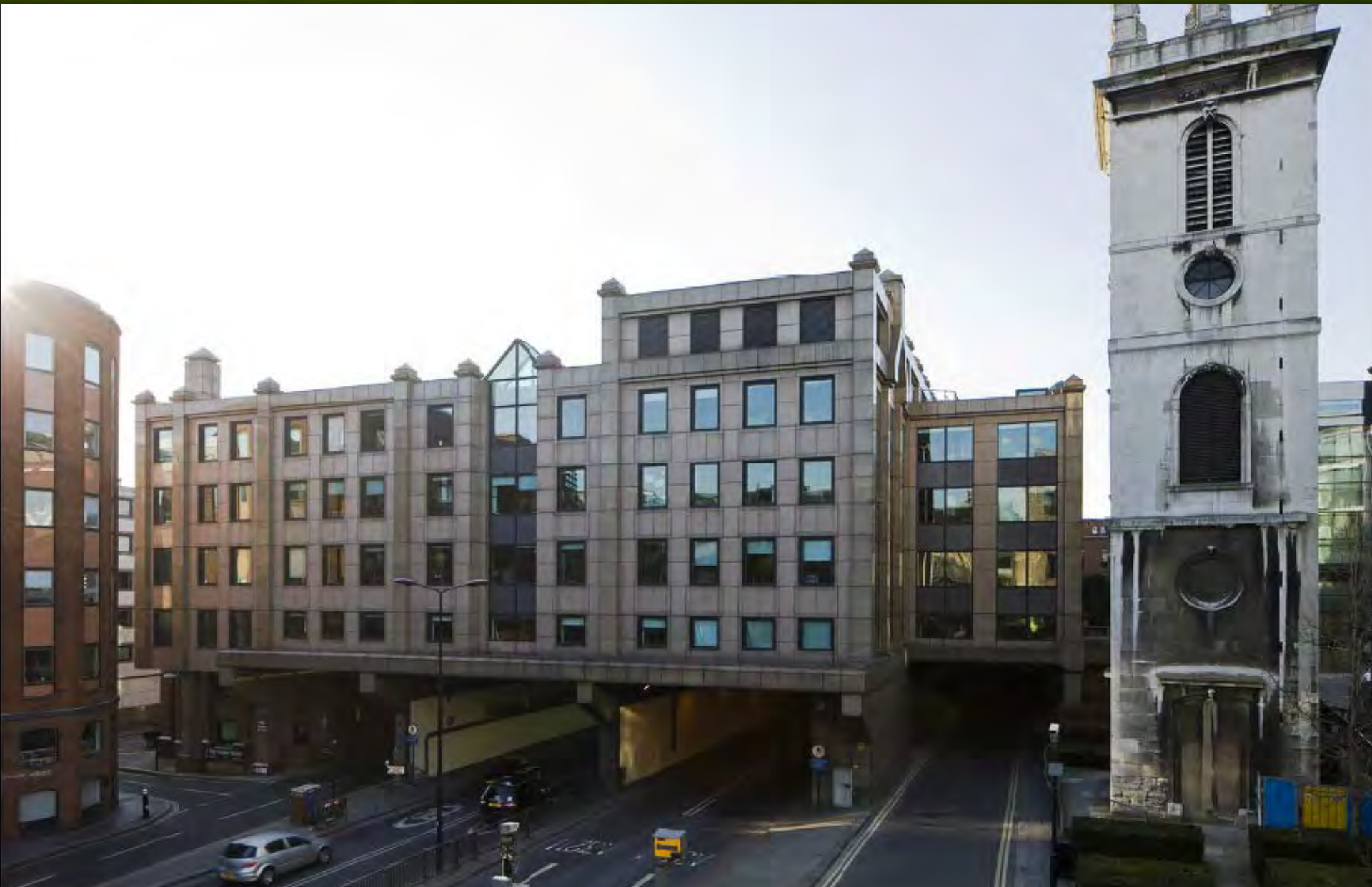
Existing view from Upper Thames Street towards St Mary's Church
